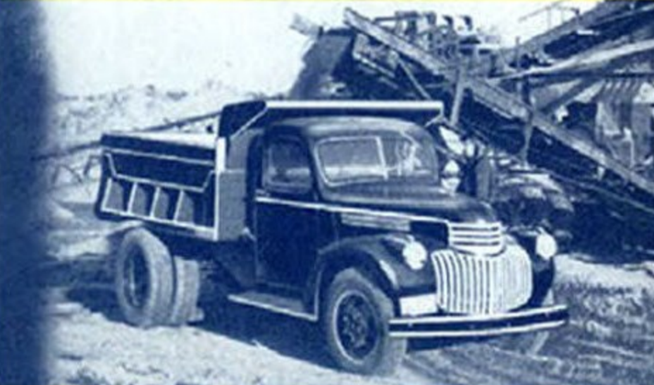
Chevrolet dump truck, three-yard capacity, 134 1/2" wheelbase.
